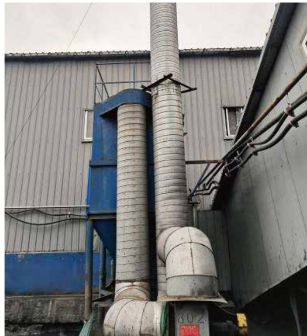
▲ Dongyu Coal Industry Bag Dust Collector
